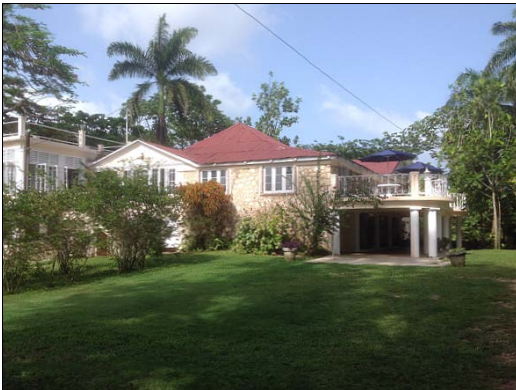
Abingdon Great House built on 1660s foundations, and the 350 year old sugar mill in its grounds.
