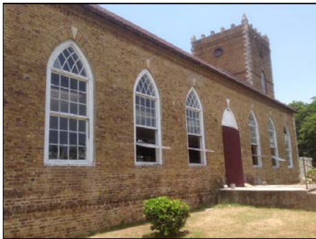
Exterior views of parish church in Black River, Saint Elizabeth, Jamaica.
