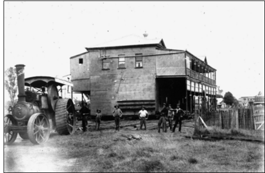
Commercial Hotel, Clermont being winched to higher ground after the 1916 flood, SLQ Neg No 18681
