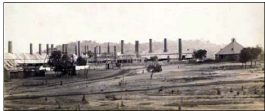
Smelting works and mine at Copperfield, Queensland, approximately 1875, by Richard James Cottell,
