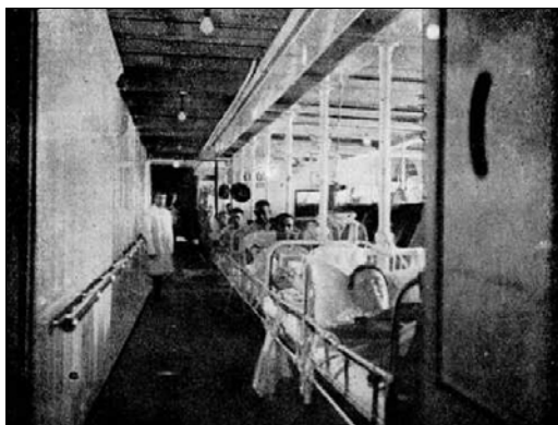
The passage alongside the ward, with space at a minimum. The Maheno's wards and operating theatres were at the heart of the ship's new role.
