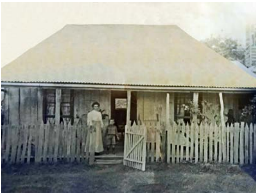
George's slab cottage, which was on the corner of Meson and Barrow Streets in Gayndah.
