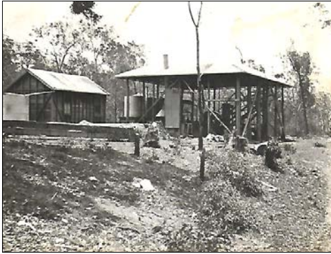
Two roomed office and machinery shed 1921 (AFC)
