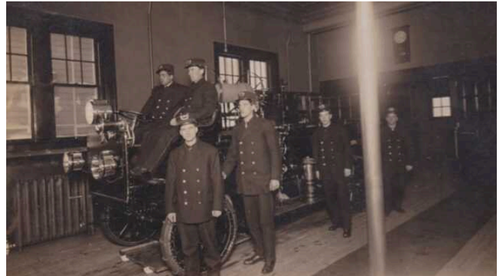
Above: Fire Hall #3, Saskatoon, c1912 [Photo courtesy of the author].
