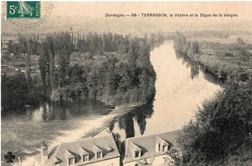
Control Dam and Vézère River dredged by contractor de la Vergne.
