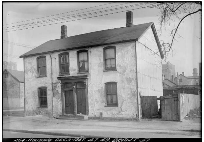
Right: 47-49 Brant Street, Toronto (Photo from the City of Toronto Archives, accessed via OldTo: Mapping Our History ( https://www.oldtto.org ).
