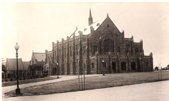
St. Peter's College Memorial Hall, Hackney Road, Adelaide, South Australia (P00170-23)
