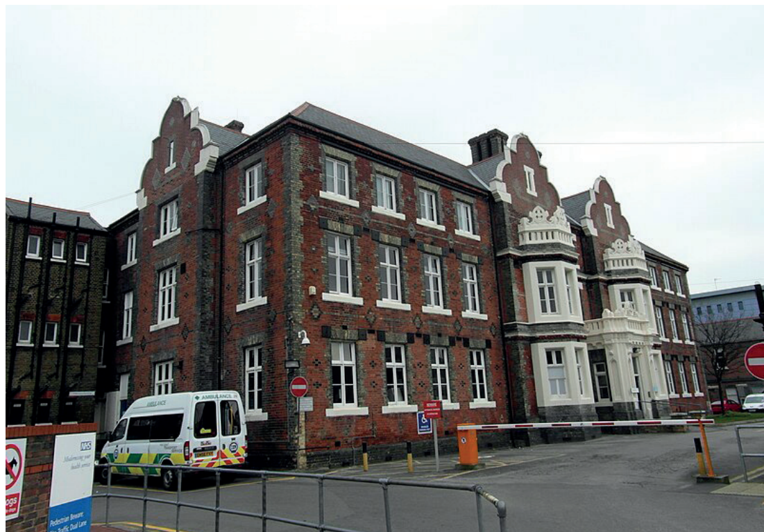
Alderney Building, Mile End Hospital in 2012. This is part of the former Mile End Workhouse, designed by William Dobson and built in 1856-8. CC BY-SA 2.0
