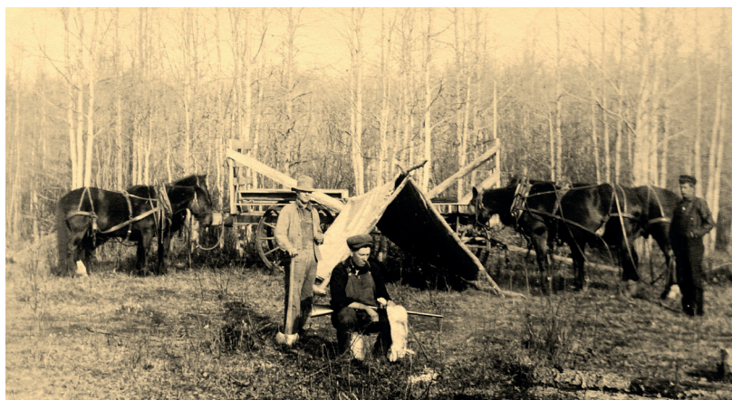
Tented accommodation in Leslieville, Samuel Turner Smith standing right
