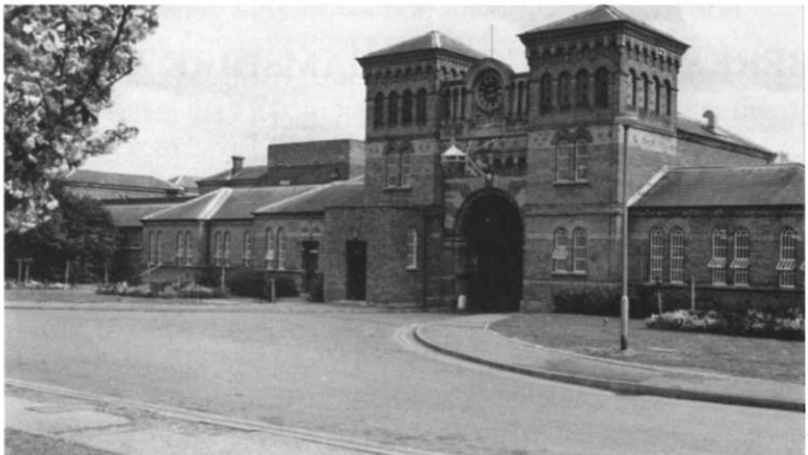
Broadmoor Old Gate
