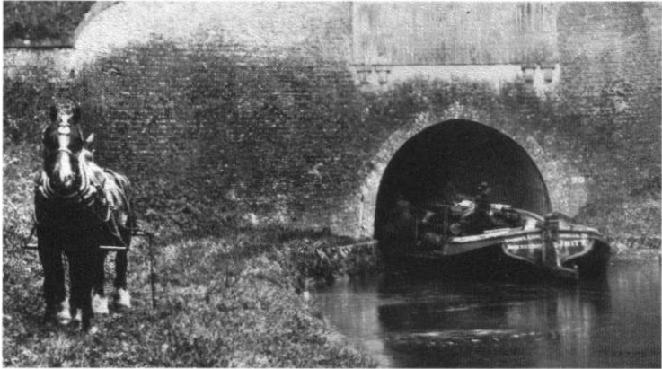
'Unity' entering the eastern portal of Bruce Tunnel at Savernake as both horses are led over the top
