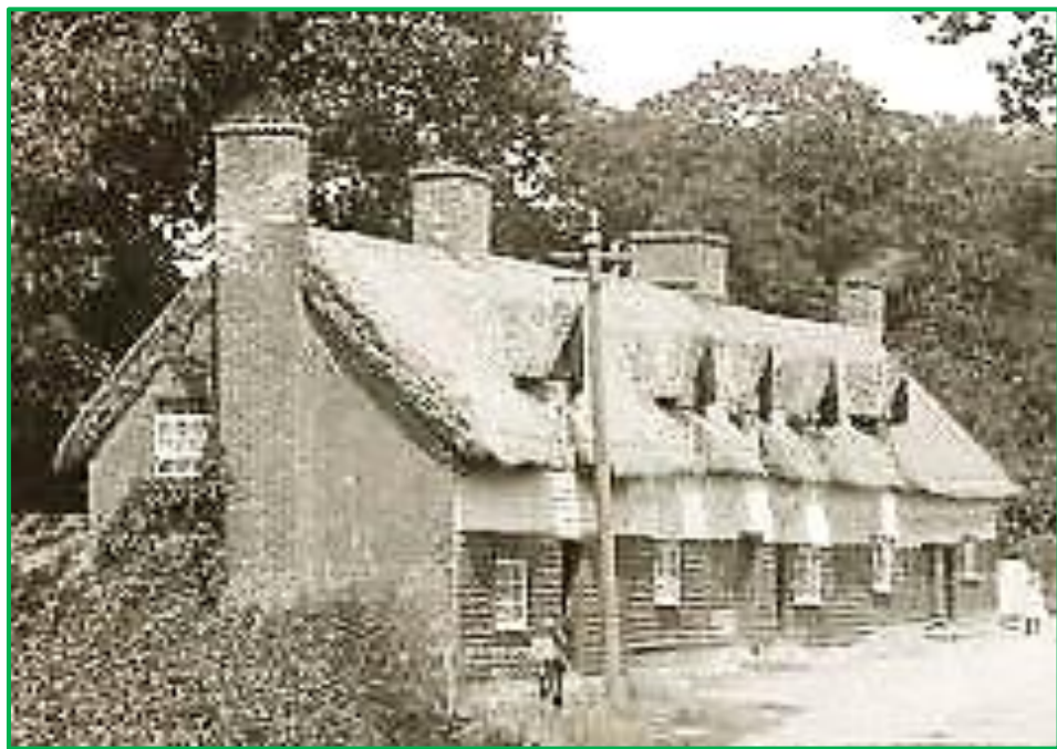
Tending, Essex parish workhouse.
