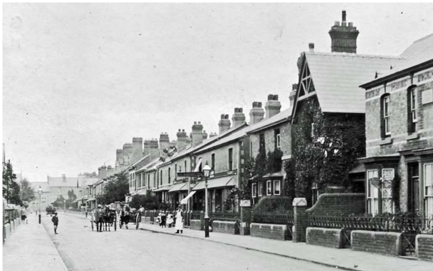
Figure 1. Chandos Street, Hereford, no later than 1907. My POWELL family were associated with three houses in the street, especially number 22, immediately right of the horses and carts. My great-grandfather Dick Powell built the house in 1893, and my grandfather and his siblings were born there. The horses and carts belonged to Thomas W. ROBINSON, grocer and milkman, of number 18.
