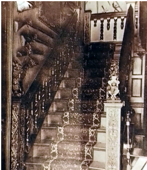
Fig.6: Interior view of the Entrance Hall of St Chad's, Uppermill, Saddleworth. Author's collection.
