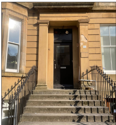
44 Kelvingrove Street - street door
