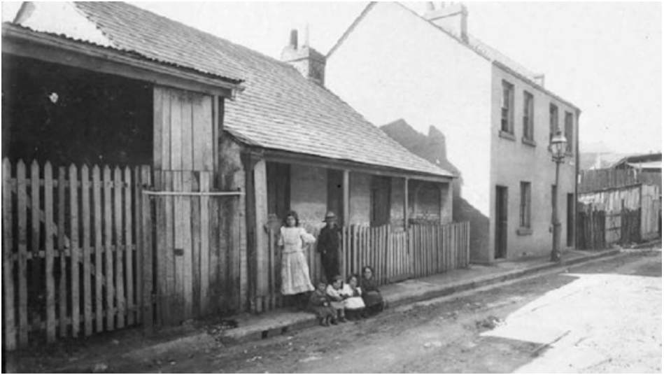
Owen Street, Ultimo in 1906 (photo: State Library of New South Wales)
