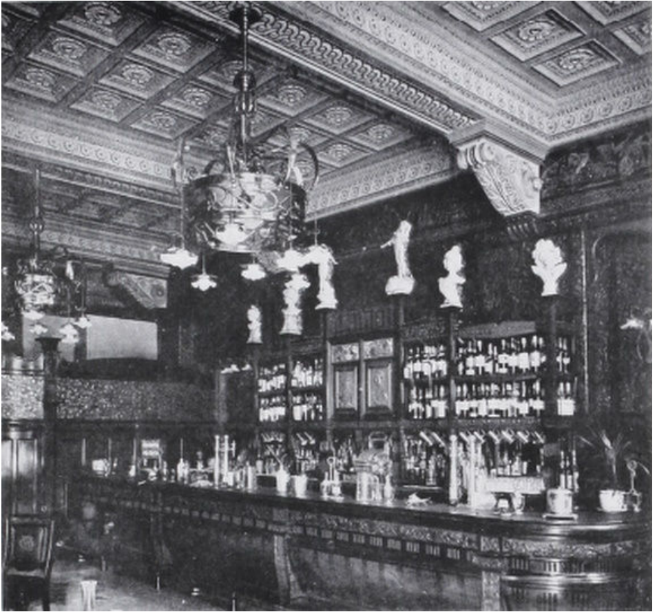
Pressed Metal Ceiling, Adam's Hotel Bar, George St. Sydney, 1888 (photo from: Forty Years of Wunderlich Industry. 1887 to 1927 , by Alfred Wunderlich)
