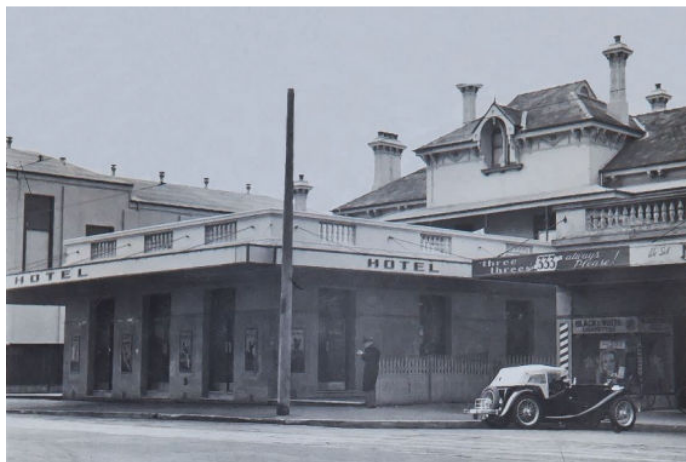
New Brighton Hotel 1949 – an ugly extension forms an entrance on The Grand Parade (photo: Tooth and Co. Yellow Cards, Noel Butlin Archives Centre, ANU, http://hdl.handle.net/1885/96620 )
