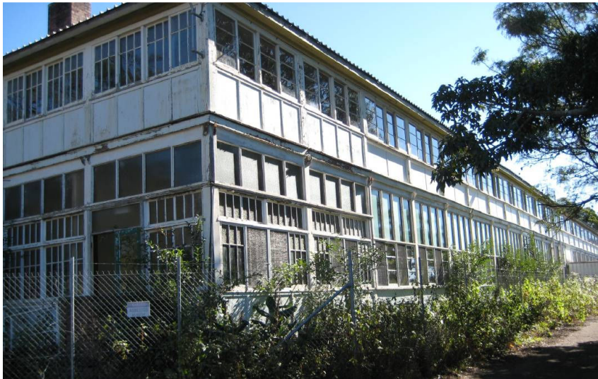
Male ward at Garrawarra, scheduled for demolition (photo: Illawarra Historical Society and Museum)
