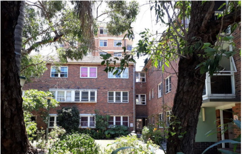
Curtin Place, corner of The Grand Parade and The Boulevard, Brighton Le Sands, designed by architects Bunning and Madden, built by C. Thompson, and named in honour of war-time prime minister John Curtin (photo: Leonie Bell)
