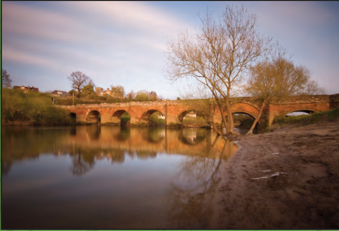
Farndon Bridge, from the west. Photo: Joopercoopers
