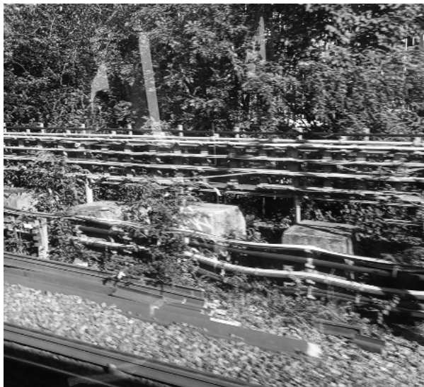
Figure 10 Anti-tank rail blocks Image courtesy of Alan Homes
