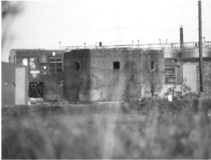
Figure 8 FW3 Type 22 pillbox at Bow Goods Yard Image courtesy of Alan Homes
