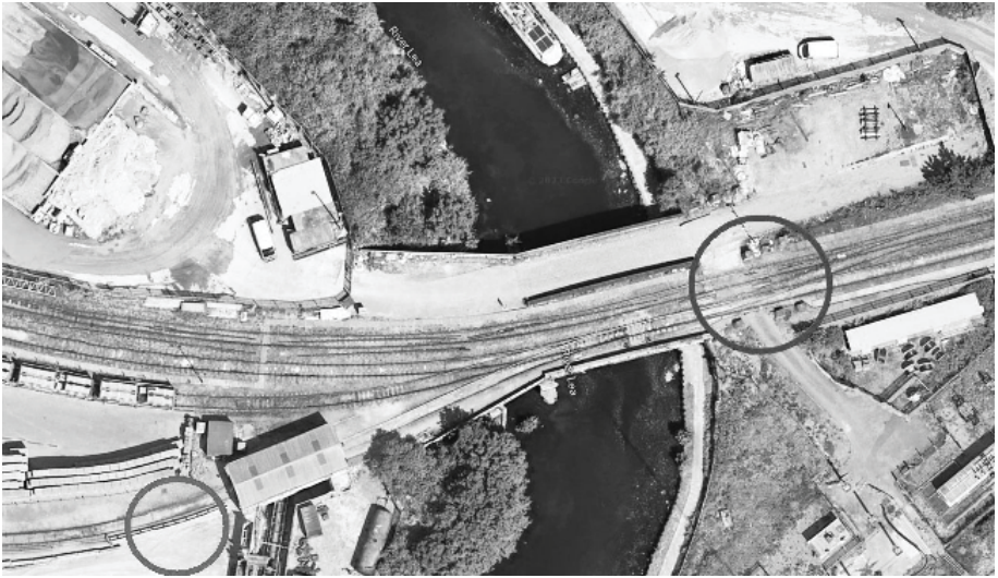
Figure 7 Aerial photo of the railway bridge
