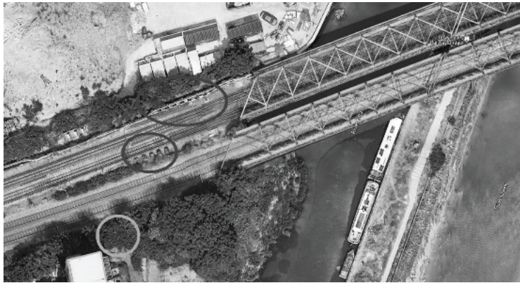
Figure 11 Aerial photo of the railway bridge across the River Lea Image courtesy of Alan Homes
