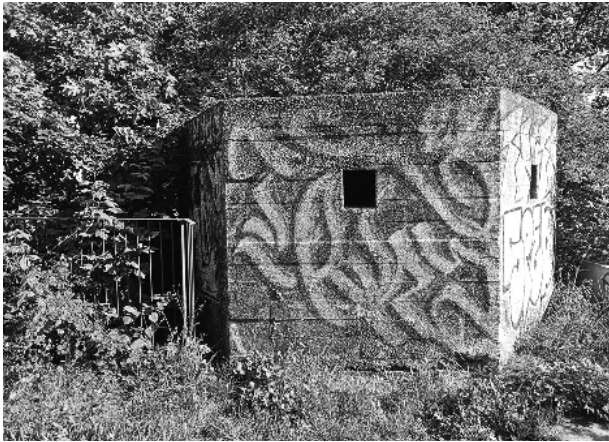
Figure 2 The FW3 Type 22 pillbox at Old Ford Image courtesy of Alan Homes
