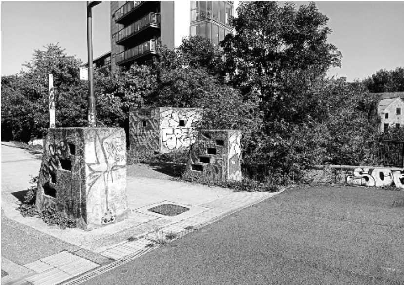
Figure 4 The FW3 Type 22 pillbox and two of the anti-tank obstacles at Old Ford (August 2023)
