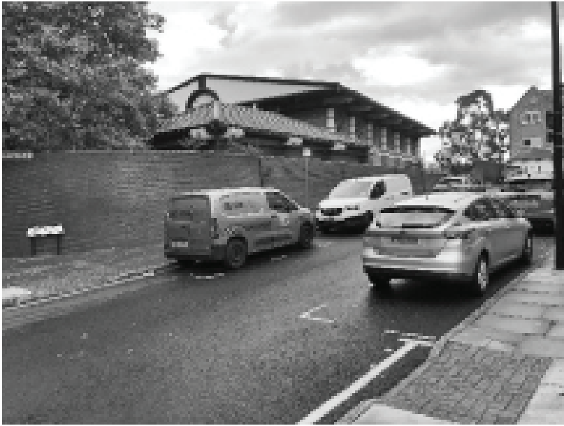
Folly Wall and the modern storm pumping station in 2022–Folly Wall is now a road running between Stewart Street and the site of the old Folly Wall at the Prince of Wales Public House
