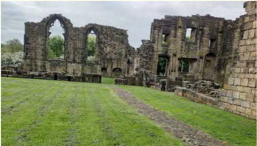
The West Window Wall with the Cloister Path on the right.
