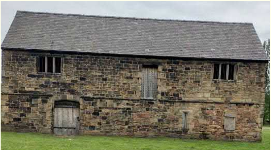
The 13 th Century Administrative Building
