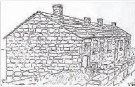
Nailshops off Towngate, Mapplewell, now demolished. From a photo taken in 1945.
