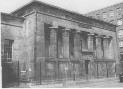
Marshall's Temple Works, Holbeck, Leeds. Only this small section of the facade was left uncovered during restoration in June 2022, the fully refurbished Marshall's Mill is just visible on the right.
