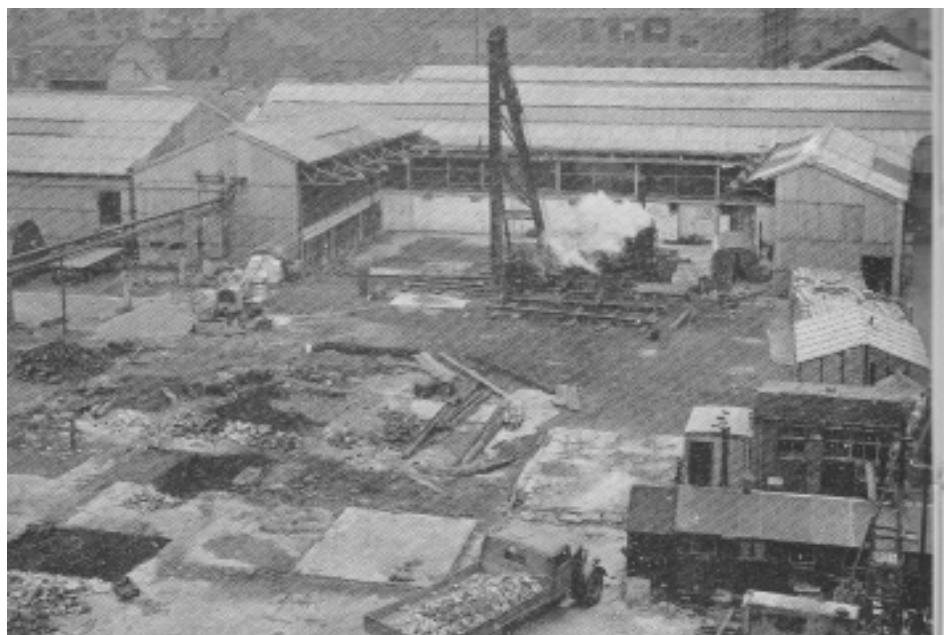
Rebuilding the Reckitts works in Hull in the 1940s
