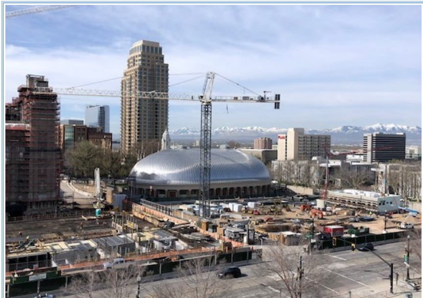
Temple Square construction, April 2023
