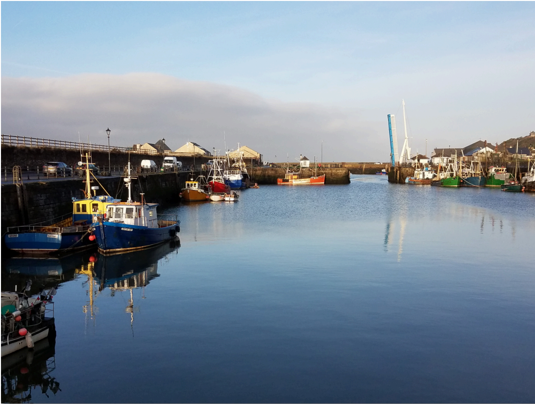
Maryport Harbour, with walkway across entrance raised to allow fishing vessels in and out. This is near high tide (author's photograph).
