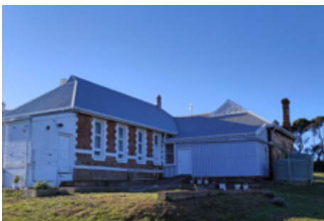
Rear view of the former Government School in Eudunda.
