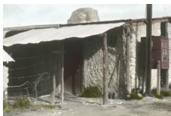
AG Burton's residence, Kilroo, South Australia, 1935 (P00197-556)
