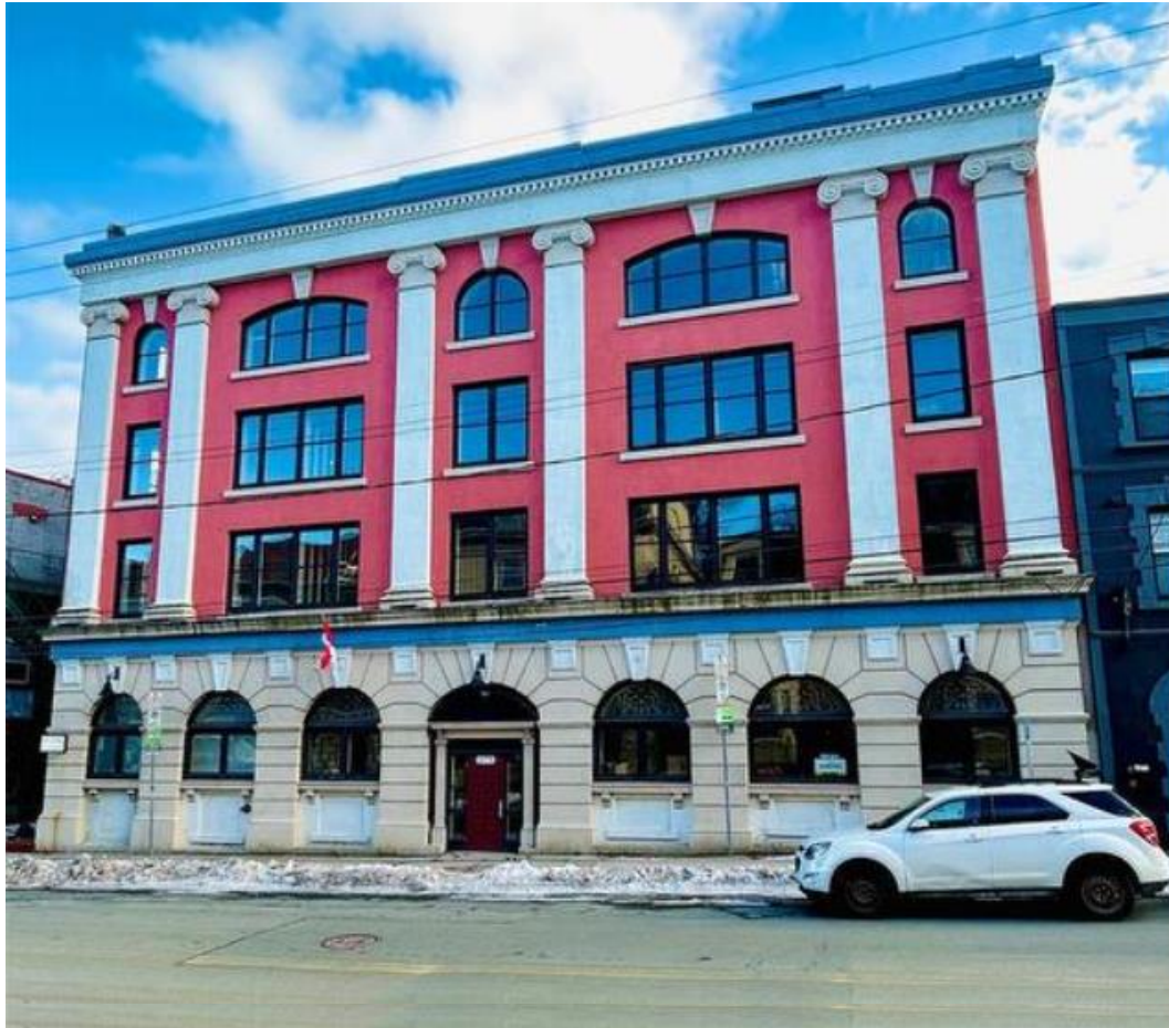
The building today at 275 Duckworth Street.
