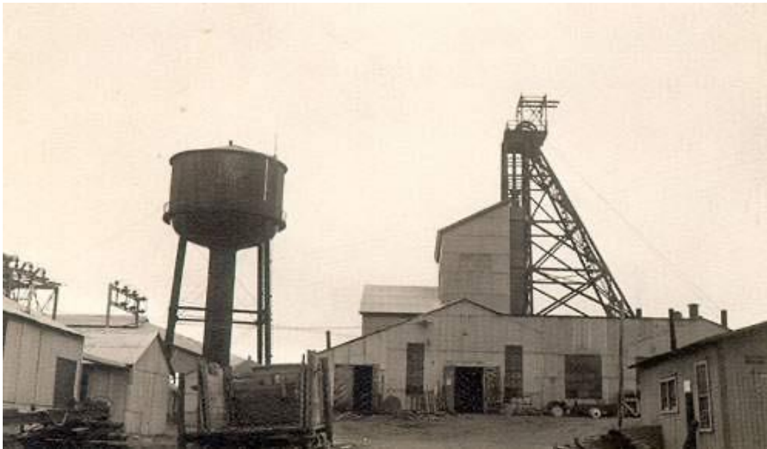
Director Head Frame and Mill Buchans Mine ca 1950 Courtesy Dept Mines and Energy
