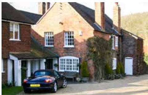
The Hale showing its older renovated brick-work at the rear, not in keeping with the facade at all. J Bateson, 2006.
