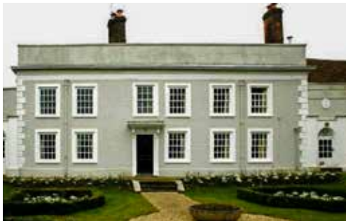
The Neo-Georgian façade of The Hale, 2006.
