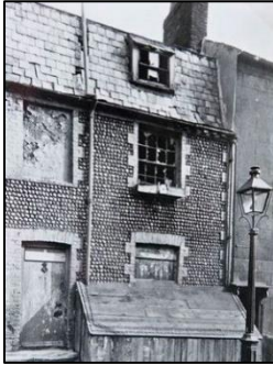
Figure 5: Old flint (beach pebble)-faced houses on John Street in 1912 (later renovated)
