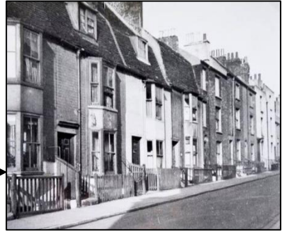
Figure 6: Old houses on John Street awaiting demolition, 1939
