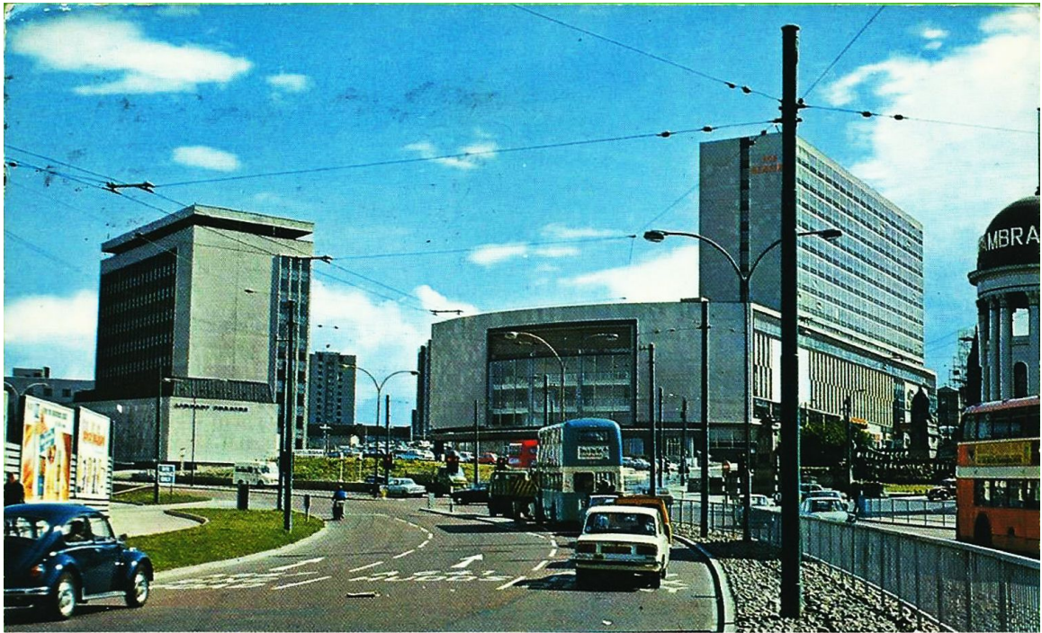
Princess Way and Central Library, Bradford
