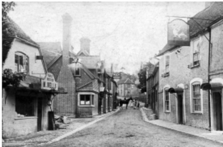
There is no record of which of the many East Ilsley inns was run by Joseph Toomer, but perhaps it was one of these in the High Street (c 1905). Reproduced by courtesy of West Berkshire Museum (1994.42)
